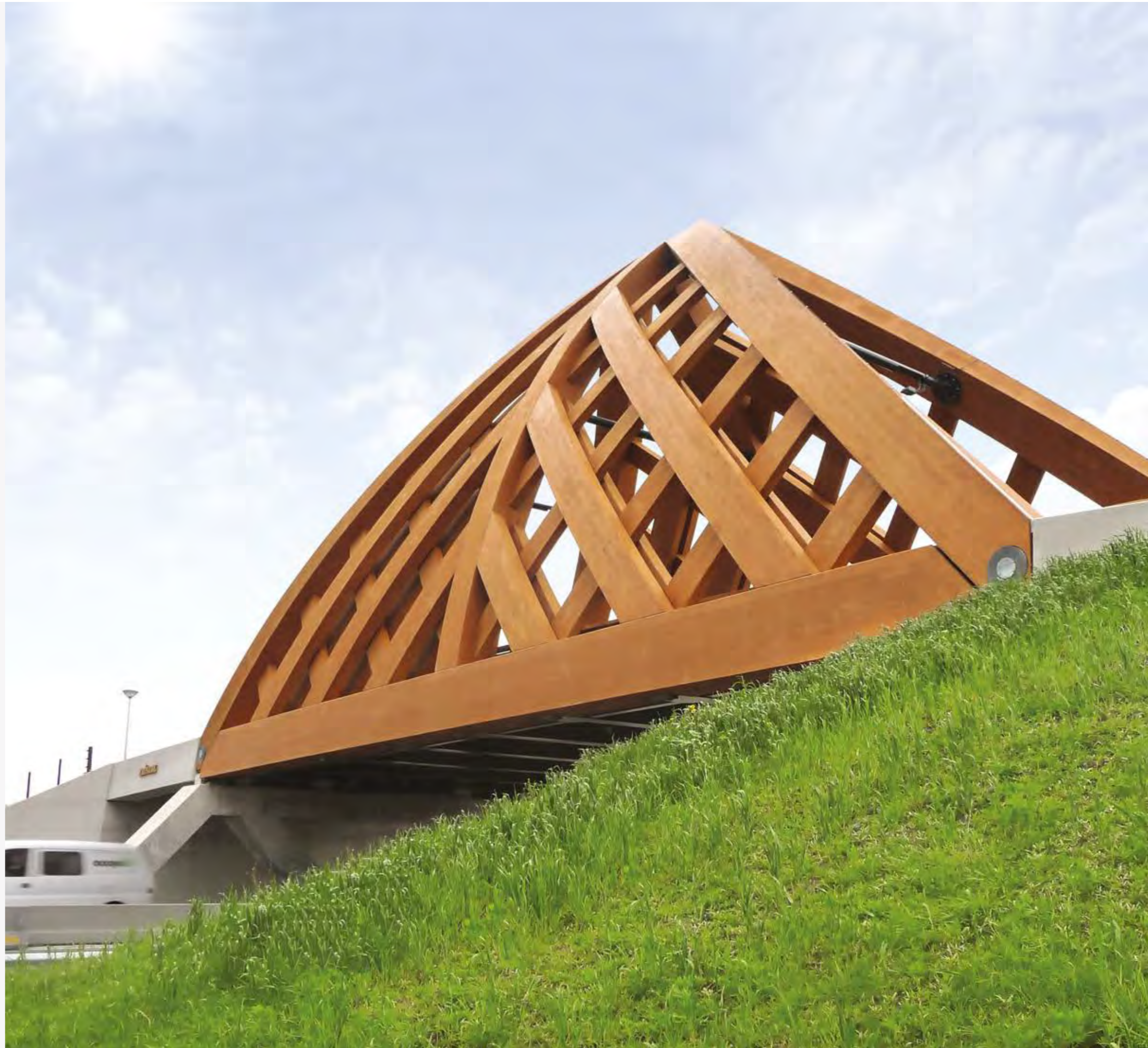
SNEEK BRIDGE THE NETHERLANDS
